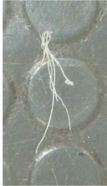
Figure 1: Scratch on the floor. Photo: MB.
