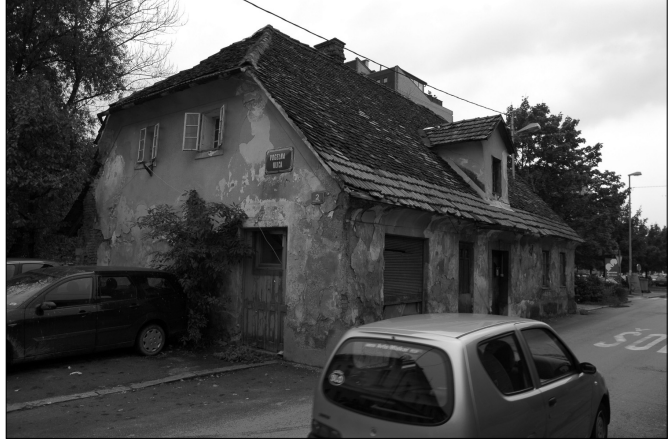
Figure 4: Trnovo historic housing [Photo: J. Fikfak, 2005].
