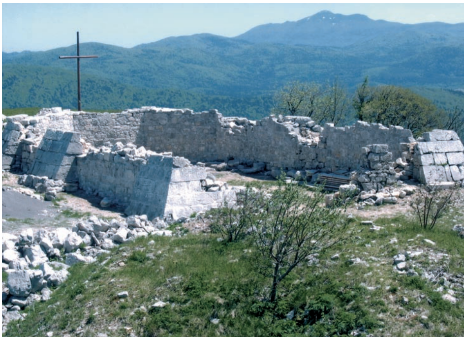
A new church is being built on the ruined foundations of the original one, on the top of Sv. Trojica.
