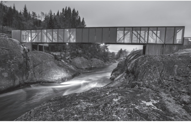
Fig. 3: An example of a gigantic joint: bridge Høse in Suldal, Norway, designed by Rintala-Eggertson Architects 2008-2013; photo by Dag Jensen.
