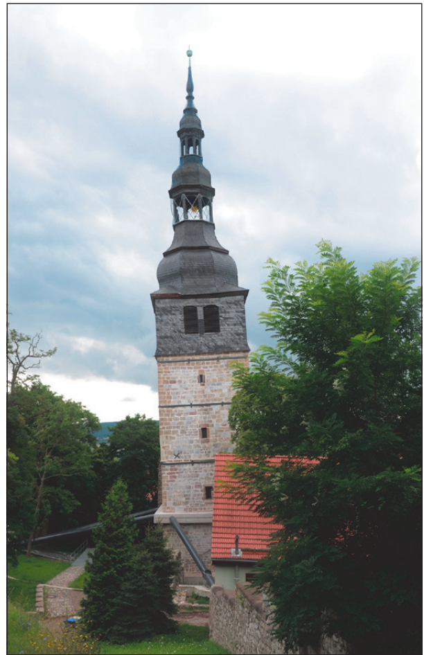
Fig. 5: Leaning church tower of the Oberkirche in Bad Frankenhausen (Photo: G. Kaufmann).
