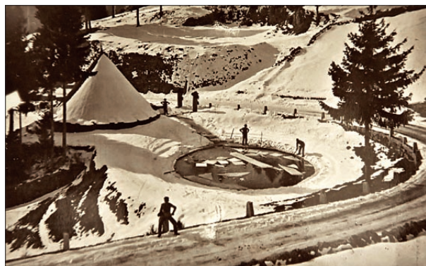
Fig. 8: Production of ice slabs obtained by the naturally frozen water small artificial lakes, then to be kept in cylindrical storehouses that were probably inspired by karst pits. The photo was taken around 1950 (Photo: unknown author).
