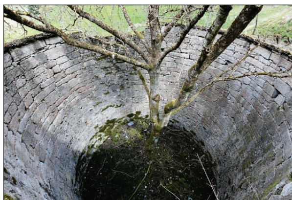
Fig. 9: The cylindrical shaft of an ice storehouse, called “ghiacciaia” or “giassara”, which was once covered with a conical roof of reeds (Photo: U. Sauro).
