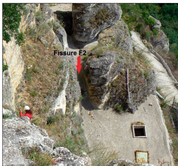
Fig. 4: The entrance of Golyamata Tsepnatina Cave (fissure F2) with the concrete roof (Photo: N. Dobrev).
