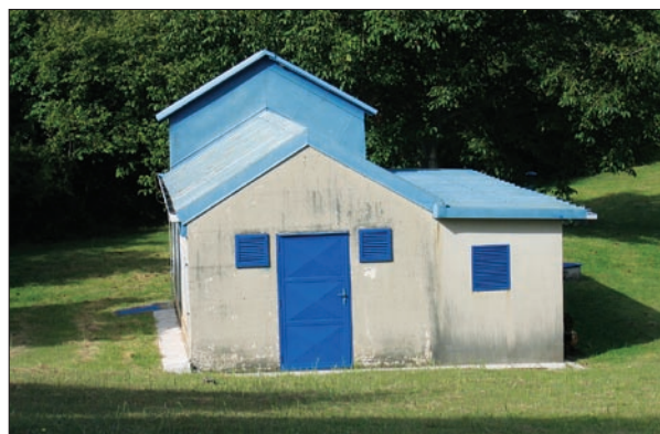
Fig. 2: Pumping station Klariči (Photo: K. Mezga).
