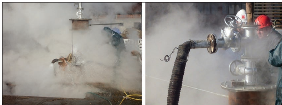
Fig. 14: Rehabilitation of well BB-1 at Bogatić (Photo: M. Lazić, 2014).
