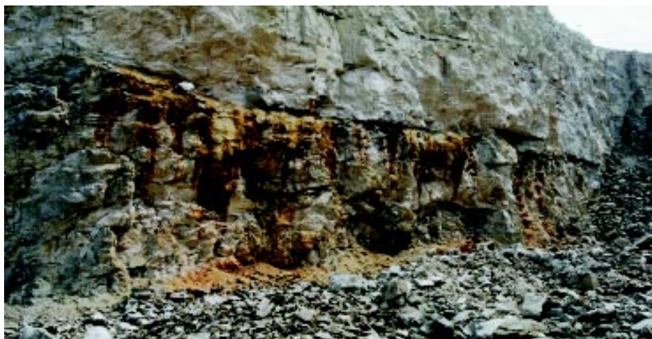
Fig. 7: A closer view of the lower face seen in Figure 6. The dominant bedding plane displays laterally extensive dissolutional voids and the rock below the bedding plane is heavily iron-stained.
