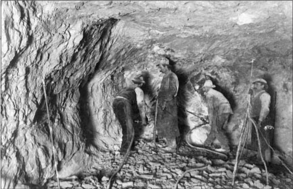
Fig. 7: Digging a carriage garage into the rock, winter of 1924/25 (Notranjski muzej Postojna collection).
