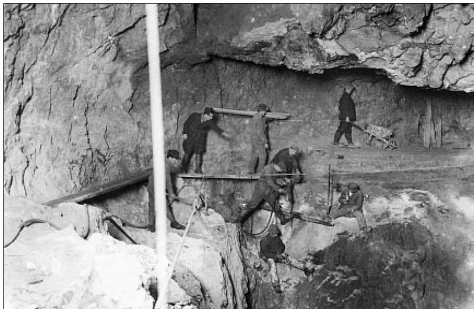
*Fig. 6: Widening of Veliki dom and levelling the ground for the railway, winter of 1924/25 (Notranjski muzej Postojna collection).*
