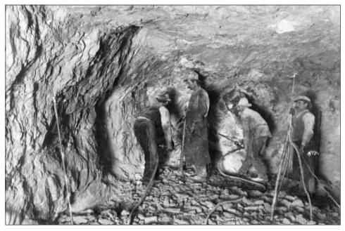
Fig. 7: Digging a carriage garage into the rock, winter of 1924/25 (Notranjski muzej Postojna collection).
