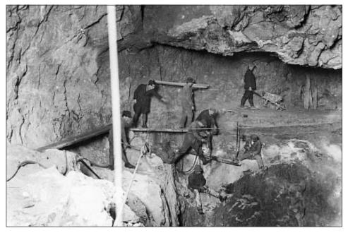
Fig. 6: Widening of Veliki dom and levelling the ground for the railway, winter of 1924/25 (Notranjski muzej Postojna collection).
