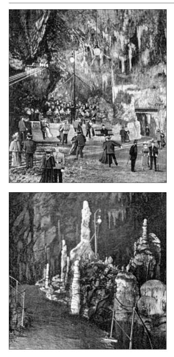
Fig. 5: A Grottenfest in what is now called Kongresna dvorana, showing two of the arc lights and their overhead wiring fitted in 1884. From a postcard used in 1903.
