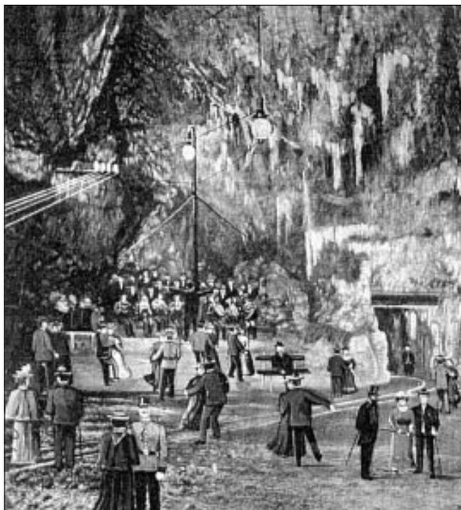
*Fig. 5: A Grottenfest in what is now called Kongresna dvorana, showing two of the arc lights and their overhead wiring fitted in 1884. From a postcard used in 1903.*
