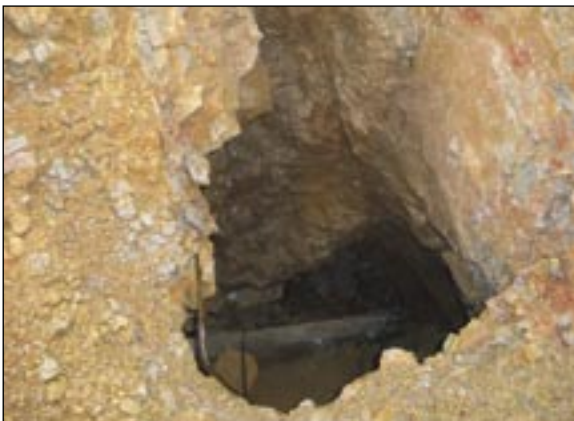
Fig. 6: The cave formed in crushed rock. Sl. 6: Jama oblikovana v pretrti kamnini.
