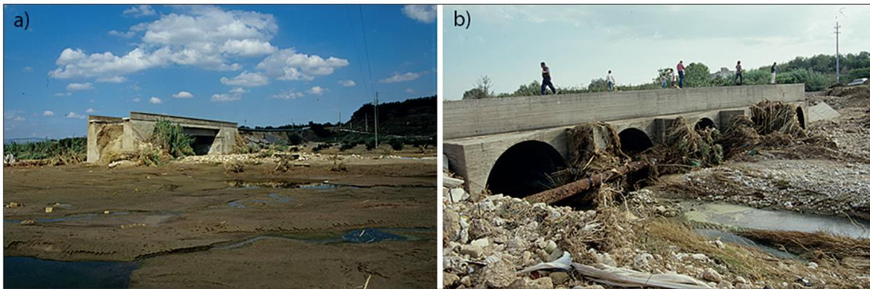
Fig. 6 – Effects of 2003 floods in karst areas in the Taranto province, southern Italy: a) road earthfill destroyed by the passage of the flood (Photo: M. Parise), and b) occlusion of bridges by trees and vegetation (Photo: M. Parise).
