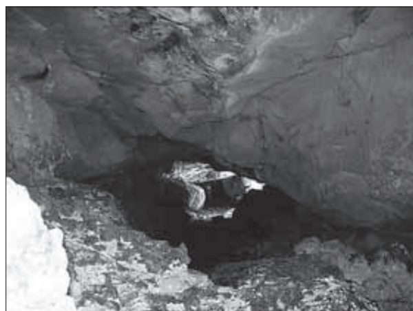
Fig. 13: Zulum overflow gallery. (Photo: A. Iurkiewicz).
