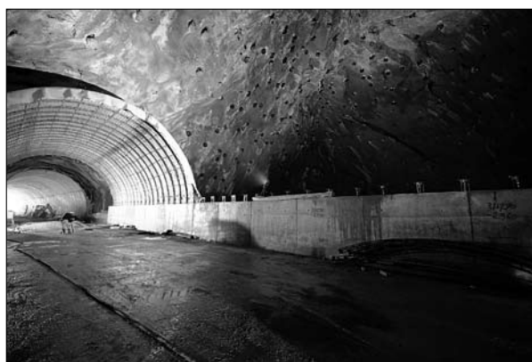
Fig. 11d: Final phase of constructing (Photo: M. Garašić).
