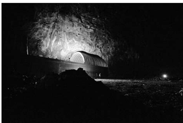
Fig. 11c: Cavern, tunnel, bridge and protecting anchors (Photo: M. Garašić).
