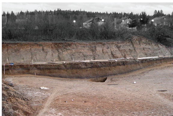
Sl. 10: Črnomelj – Svibniki, stratigrafija na območju arheoloških izkopavanj 2009 na trasi črnomaljske obvoznice. Fig. 10: Črnomelj – Svibniki, stratigraphy in one of the swallow holes during the archaeological excavations in 2009 in advance of the construction of the Črnomelj Bypass.
