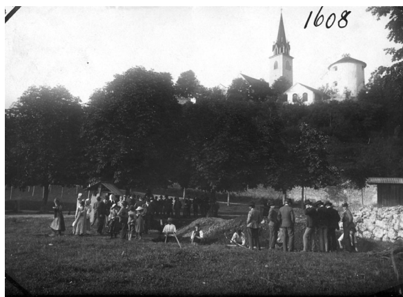
Fig. 5: Photo 1608. Lajh underneath Kranj. Excavations of 1901. View towards the northeast with the church of St Roch in the background.
