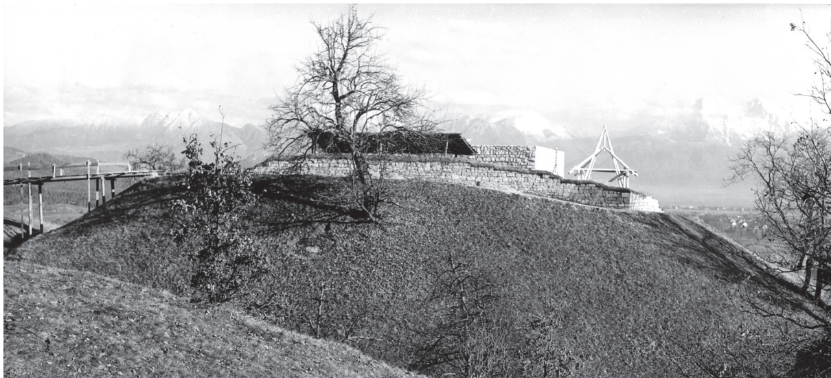
Fig. 6: Krancelj above Škofja Loka. In situ presentation of the excavated remains of the so-called Upper Tower in 1955 (Loški muzej; photo: T. Mlakar).
