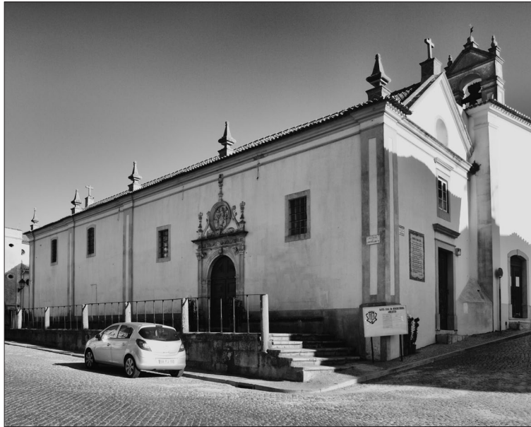
15. Exterior facades, 1548, House of Mercy, Abrantes
