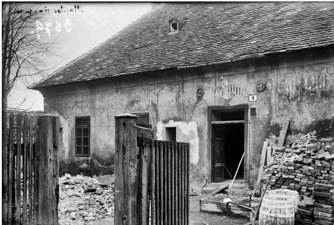
10. France Stele's photograph of the northern facade of Maribor synagogue during the renovation works in 1926
