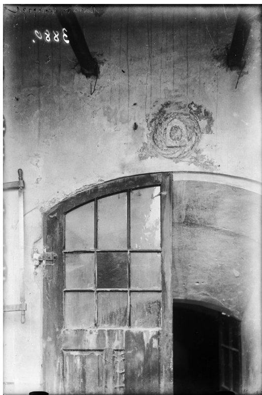
11. Keystone with a motif of grape, basement entrance at the eastern façade of Maribor synagogue
