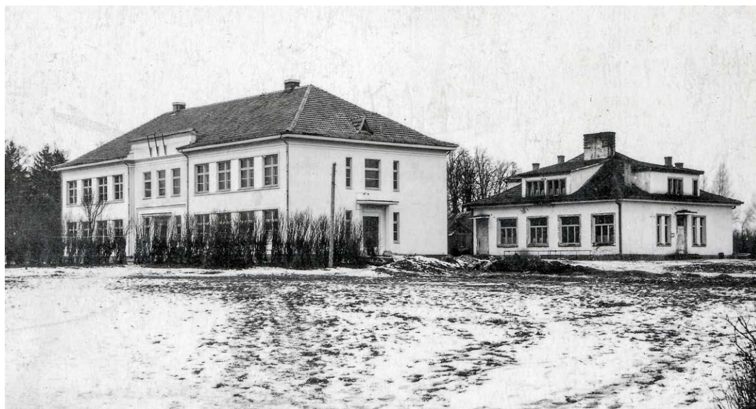
7. Šakiai County Hospital on the left, by the engineer and architect Nikolajus Mačiulskis, 1934, and the auxiliary building on the right, by the civil technician Vincas Puskunigis, 1935, photographed in the 1950s (author's personal collection)
