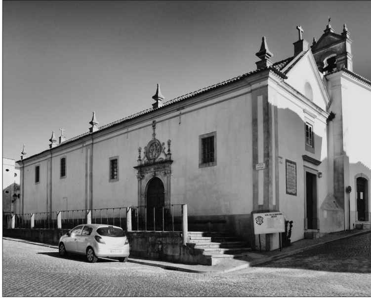
15. Exterior facades, 1548, House of Mercy, Abrantes
