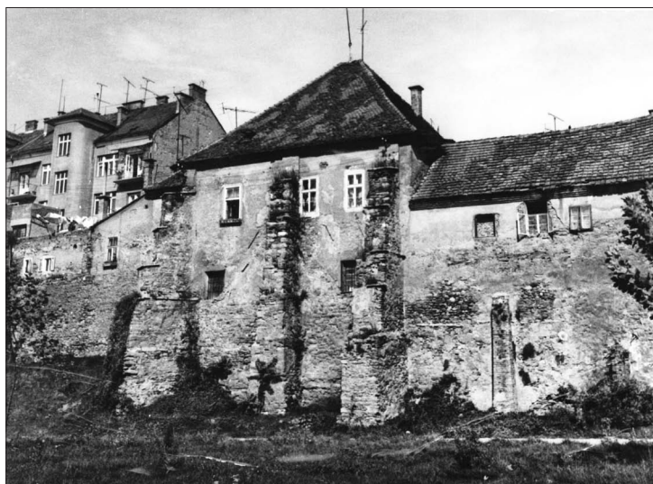
20. Southern façade of Maribor synagogue, the state before the 1992 renovation
