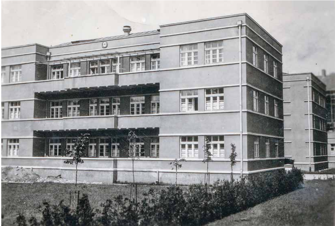
4. Southeast façade of the Lithuanian Red Cross Society's hospital in Klaipėda, photographed in the 1930s, by the engineer and architect Romanas Steikūnas, 1932 (author's personal collection)
