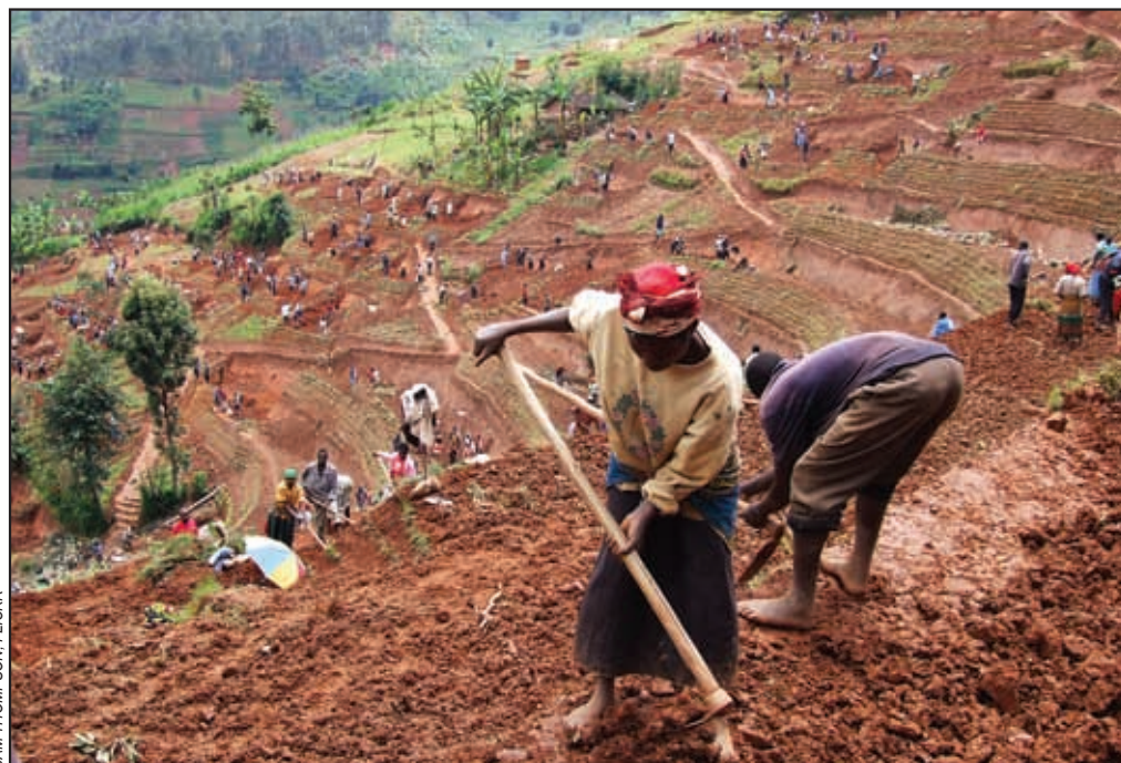
Figure 10: Terracing a slope in Rwanda as part of public works.
