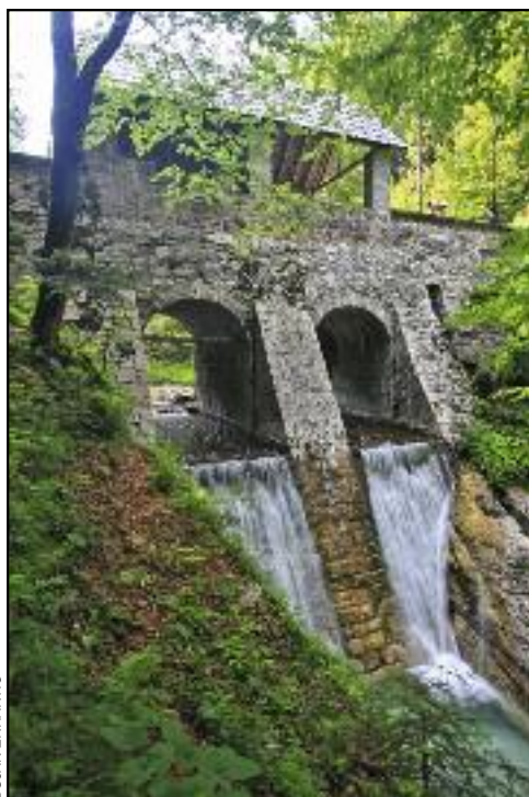
Figure 4: Logging sluices are also part of world heritage. The photo shows the Brus sluice (also known as the Belca sluice).
