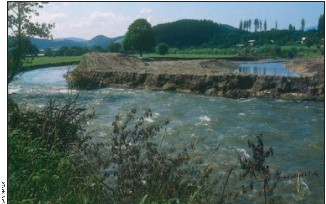
Figure 13: Right – the old riverbed in which the remaining bigger pebbles are visible, after the smaller particles were swayed away by the flood. The new regulation moved the river into the old bed.
