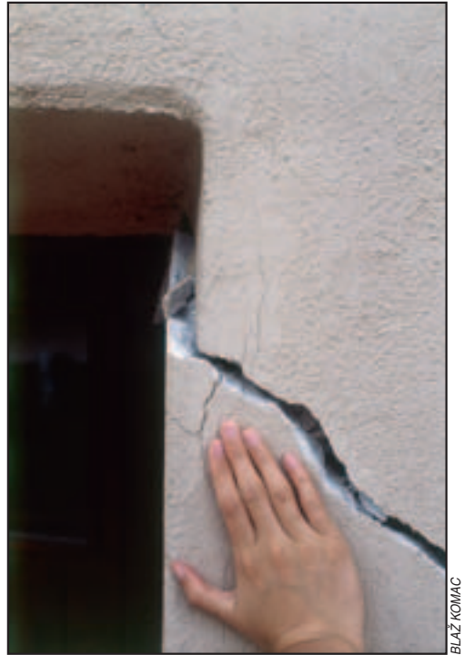
Figure 1: Buildings' corners are most critically affected in earthquakes (aftermath of an earthquake in the Upper Soča Valley)
