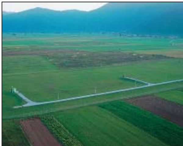
Brest water pumping station (photograph: Aleš Smrekar). Vodarna Brest (fotografija: Aleš Smrekar).
