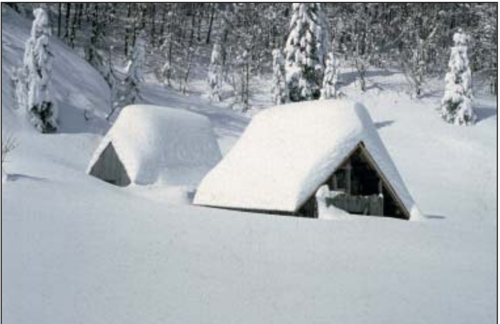
Figure 3: The Ravne alp on 27 th March 2004 (photograph: Matej Ogrin).
