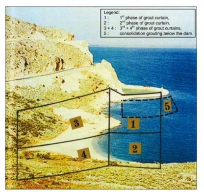
Fig. 16: Kivery dam. Desalination structures proposed (2008, photo Breznik 1969).
